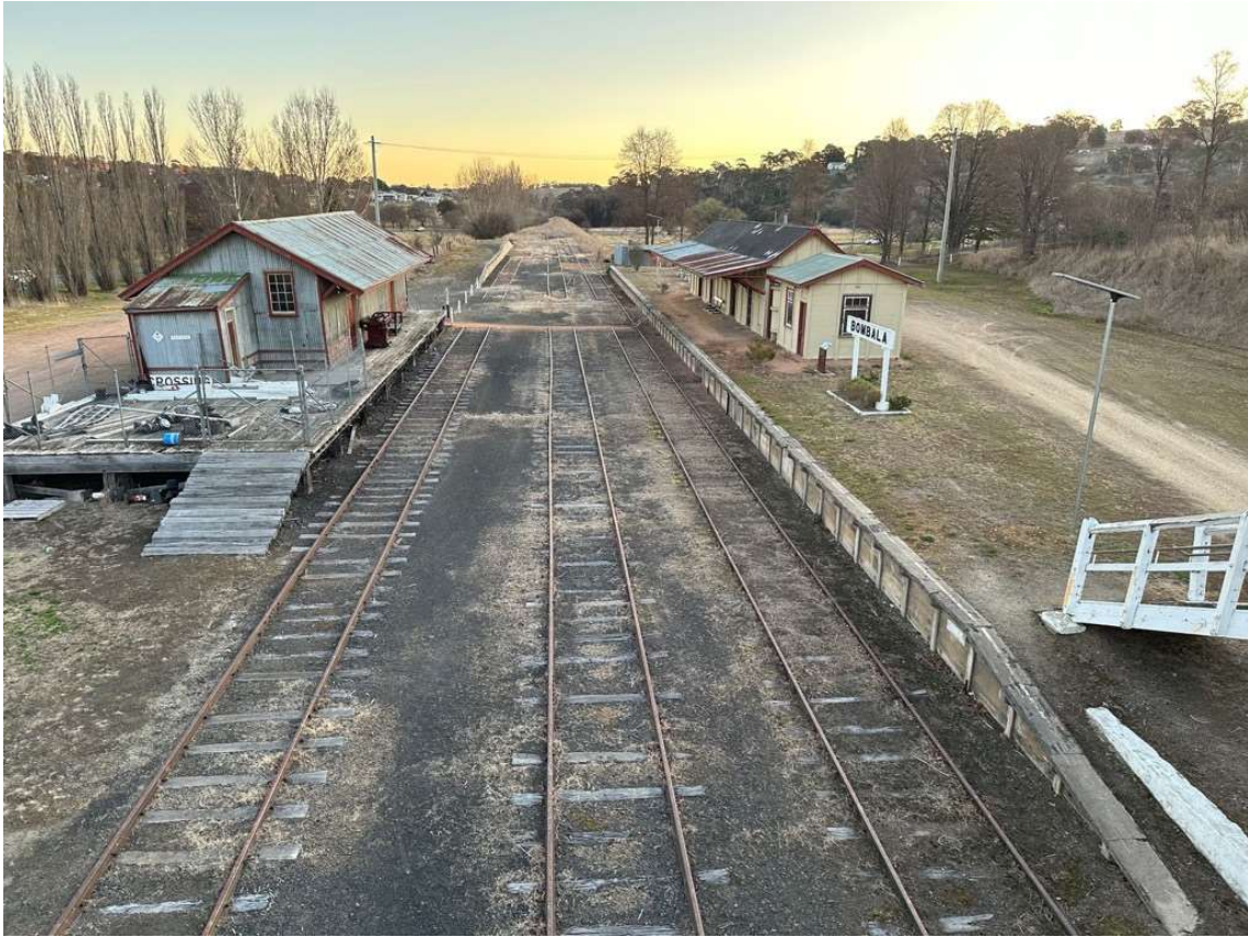
Dis-used Bombala Railway Station and precinct (leased by SMRC)
