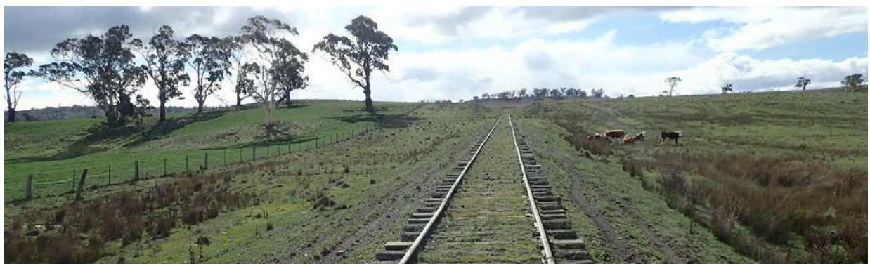
Much of the disused railway corridor would need new fencing. Some parts have fencing one side; much of the corridor has no fencing. This would be a major cost component of developing the trail.
