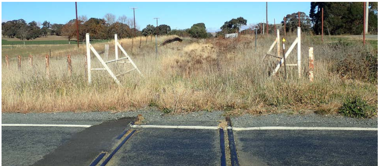
Approximately 40-45 roads cross the disused railway, including this crossing at Williamsdale.
