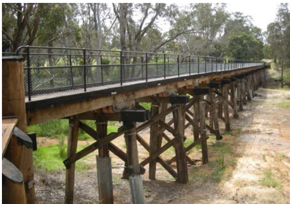
Above: The Sidings Rail Trail (WA) makes the most of existing historic rail infrastructure. This trail has two elements – as well as being a rail trail in itself, it is part of the Munda Biddi Trail – the long distance mountain bike trail between Perth and Albany.
