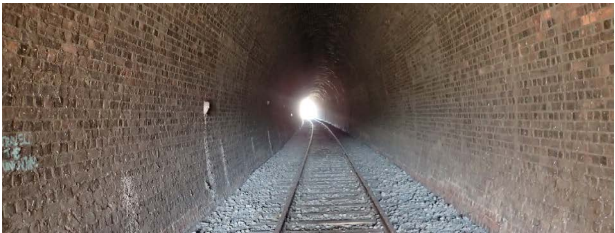
Brickwork within the Colinton Tunnel appears to be in excellent condition, although its structural integrity should be assessed prior to development of the proposed rail trail.
