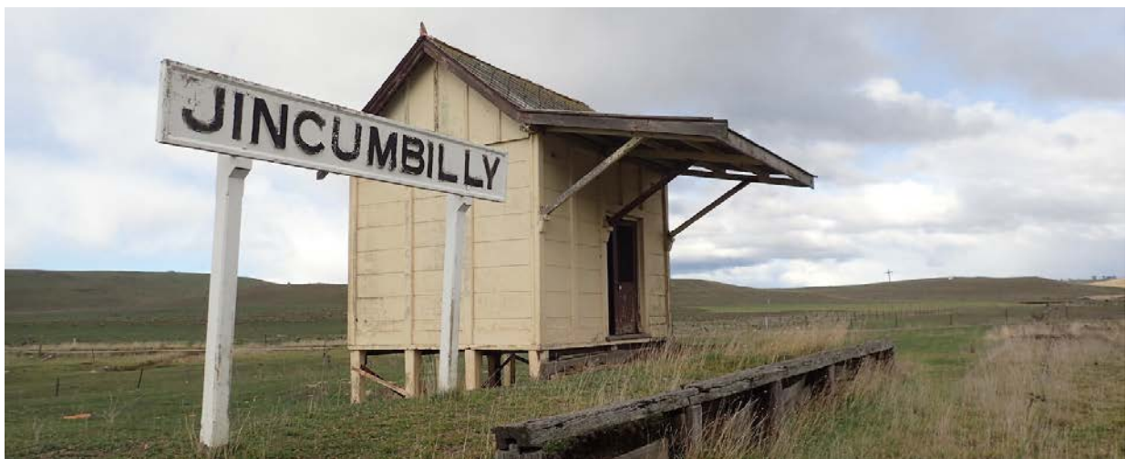
The siding shed at Jincumbilly would provide an excellent shelter in times of inclement weather. It would also provide a suitable framework for a toilet within the trailhead development.
