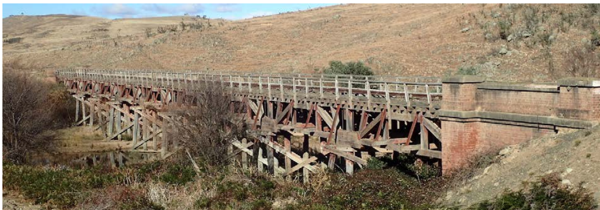
The bridge over the Bredbo River is very attractive, historic and a prominent feature of the proposed rail trail.
