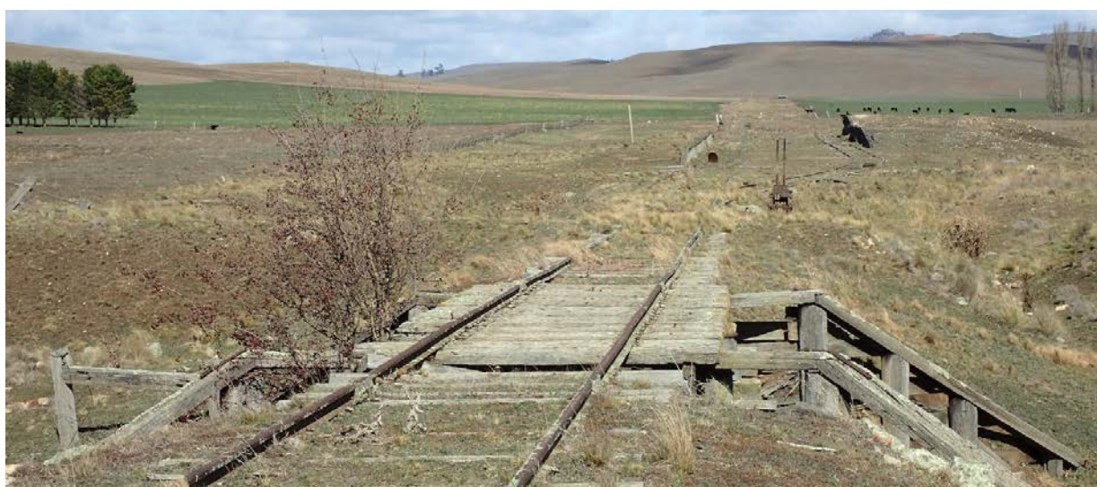
Elements of the remaining infrastructure include bridges, sidings, switches and, in some locations, the original stations, signals and distance pegs.
